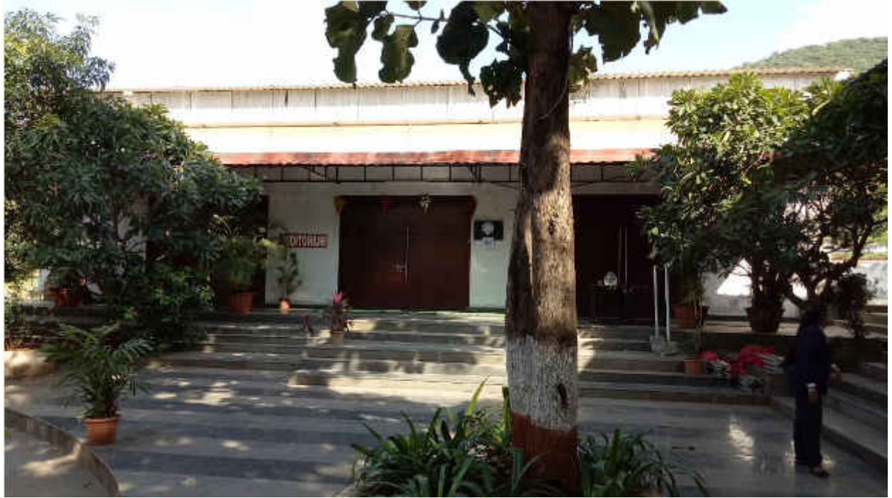
ISB&M SCHOOL OF TECHNOLOGY –AUDITORIUM
